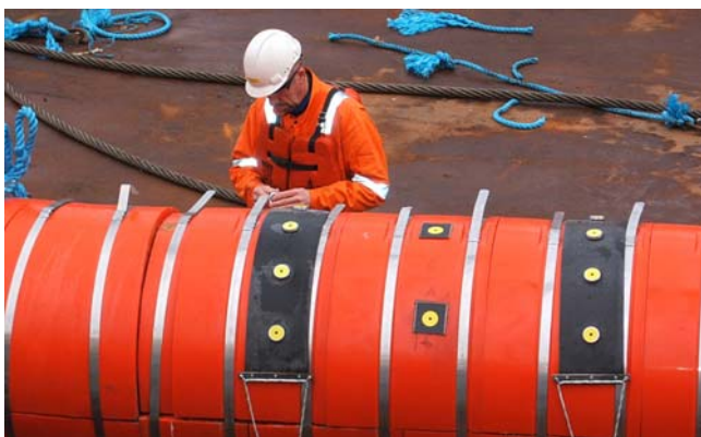
Image 2 - Rubber target mats and two survey control targets shown attached to the spool
